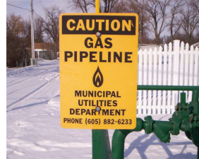
Example of a natural gas pipeline marker.
