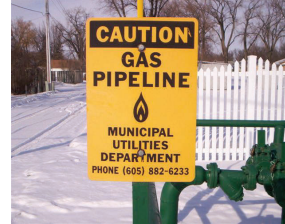
Example of a natural gas pipeline marker.
